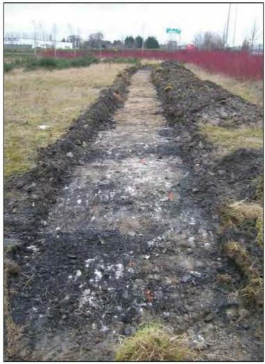
Plate 8 - Detail of modern road surface identified within Test Trench 1, Sub-area 16.
